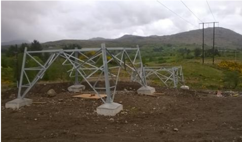
Plate 2.2: A 110 kV interface mast foundation complete
