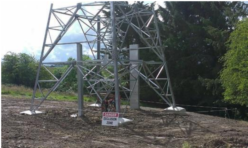
Plate 2.3: Base of an interface mast structure backfilled
