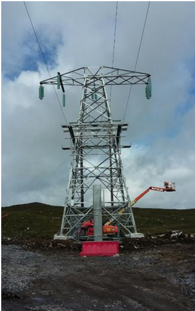
Plate 2.4: A completed line/cable interface mast
